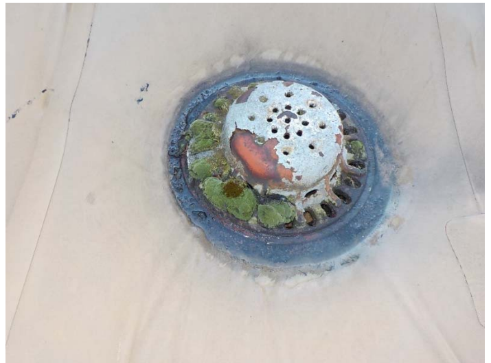
View of vegetation in roof drain.
