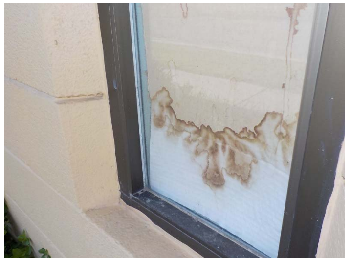
View of typical single pane window.
