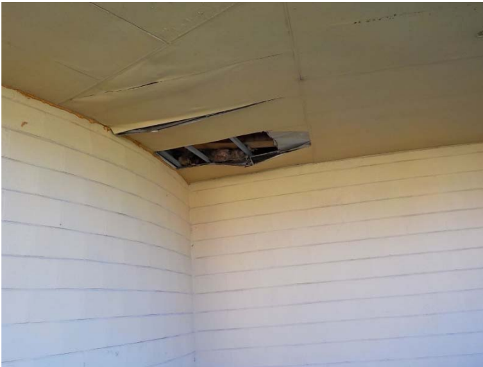
View of damaged wood soffit and insulation.
